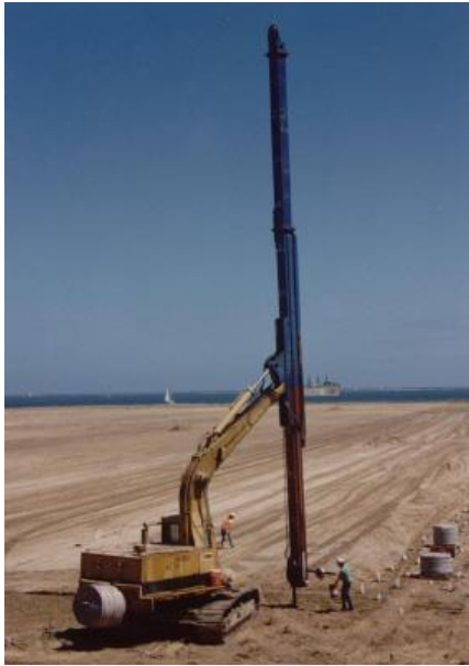
(a) Adapted Pile Driving Rig (compl. American Wick Drain)
