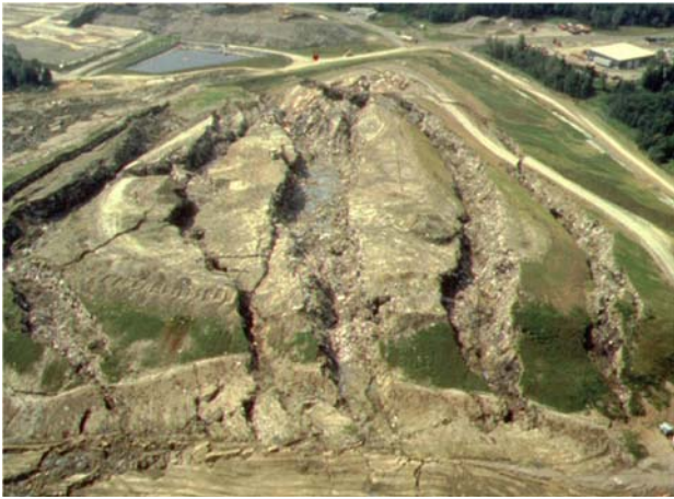
(a) Multiple rotational failure (500,000 m 3 )
