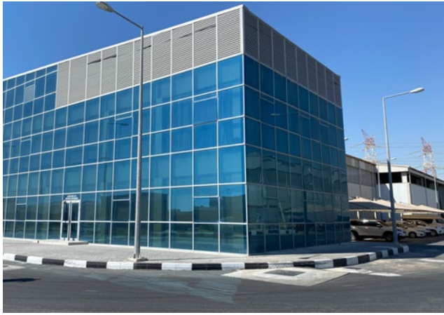
Photo outside of DWF's lab
