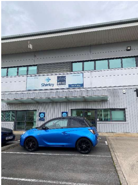
BTTG Facilities in Manchester
