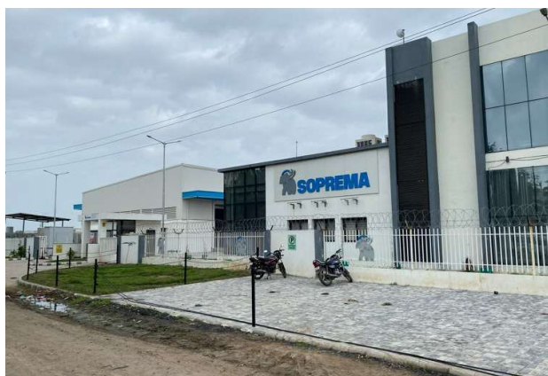
Photo outside of Soprema's lab
