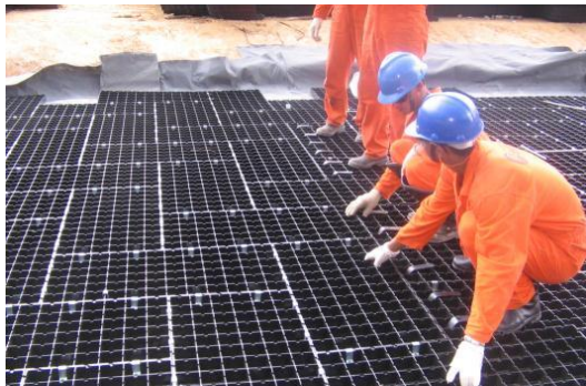
( a ) Well pad protection
