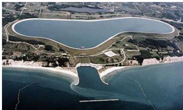
Figure 8. Concept and example of pumped-storage method of generating hydroelectricity (compl. U. S. Bureau of Reclamation)
