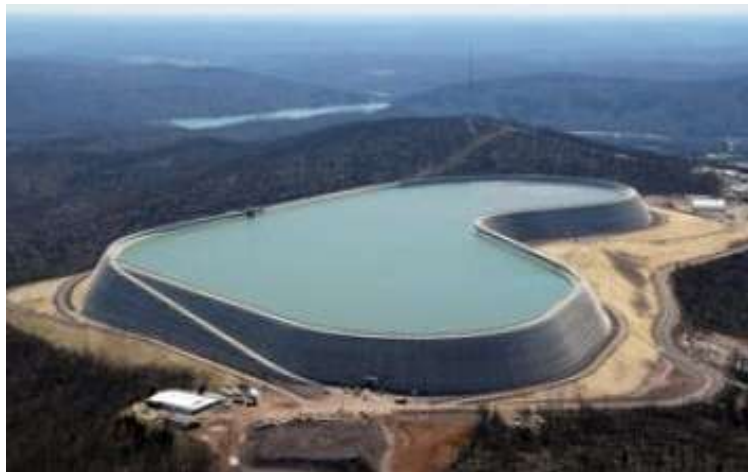
Daytime: Water flows downhill through turbines, producing electricity
