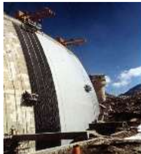
(b) Concrete dam
