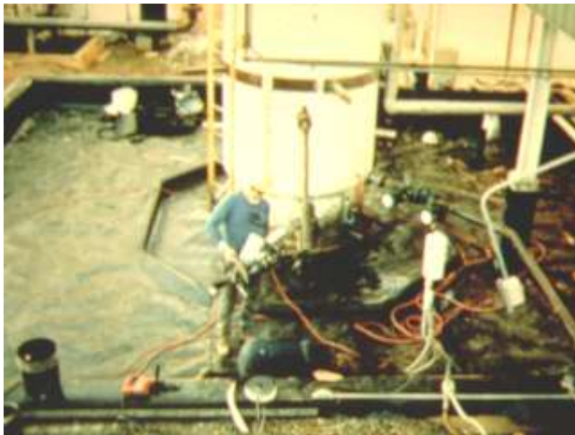
Figure 3. Geomembranes used as secondary containment for tank farms, gas stations, etc.
