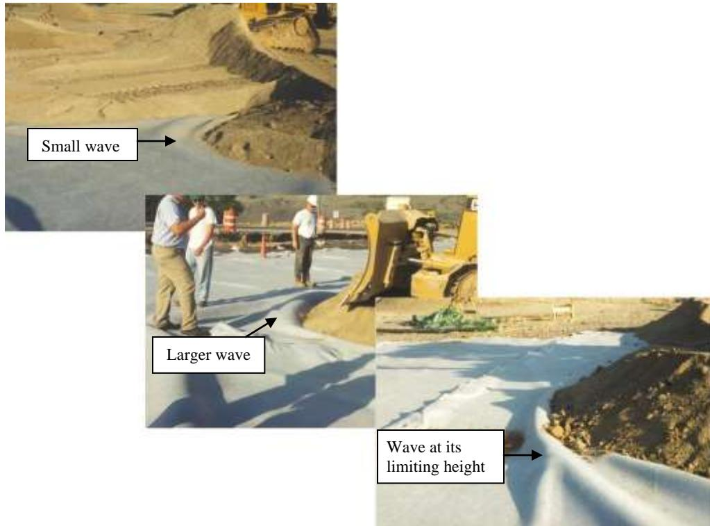
Fig. 8 – Push/Accumulate/Cut/Seam method to achieve intimate contact (compl. B. Smith).
