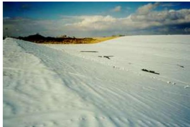
(b) Co-extrusion white surfaced sheet
