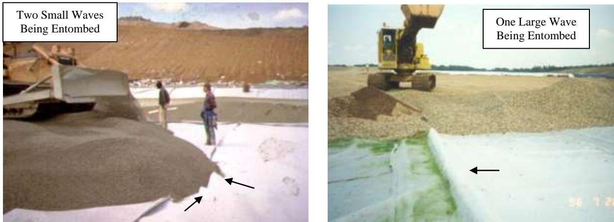
(a) Waves being entombed during backfilling
