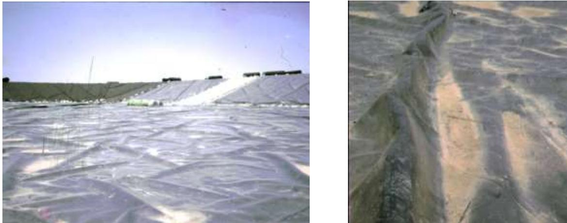
Fig. 1 – Waves in exposed geomembranes (GSI photos).
